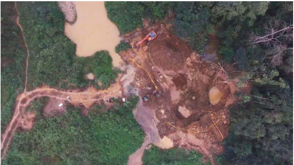
Destruction from illegal mining meted out on the Atewa Forest. Photo Credit- A Rocha Ghana
